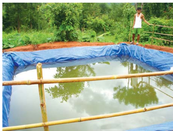
Fig 20. A Jalkund filled with rain water in Umsaw Khwan made as a part of SWPAL demonstration
